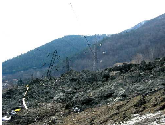
Fig. 5. Massive ground slide that damaged 110 kV and MV overhead lines
