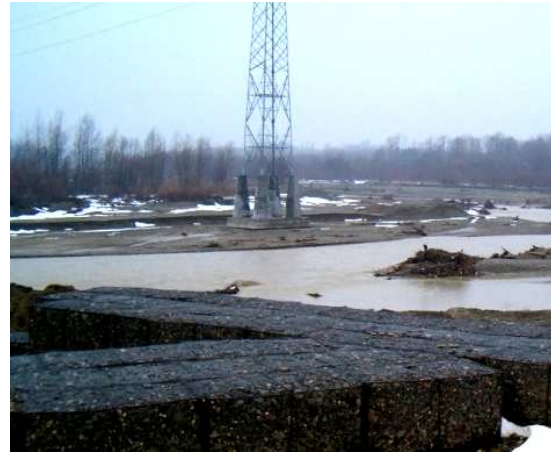
Figure 8. Benoto piles and river bank consolidation
